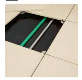
For raised installation, slabs are installed onto supports with a distance of 3mm between adjacent slabs once the underlying footing has been duly layered with water-proofing materials. In this way, there is a technical gap below the foot-plan that can be easily inspected by lifting the slabs.
